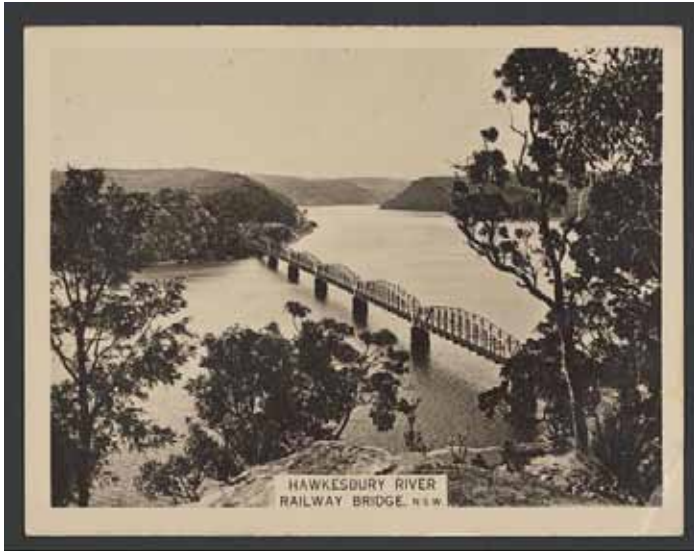
Hawkesbury River Rail Bridge 1925
